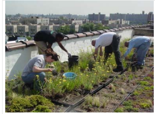
Figure 21: BEST Green Job Training participants install a green roof. Majora Carter Group
