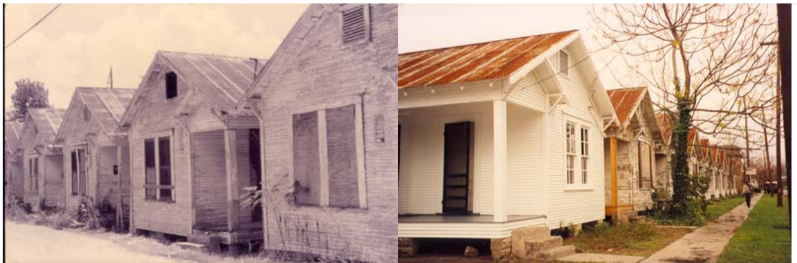
Figure 19: Shotgun houses of PRH historically (left) and with one restored (right). Project Row Houses
