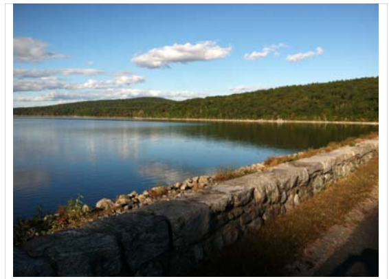
Figure 24: Goodnough Dike at the Quabbin Reservoir. Galaski, 2013
